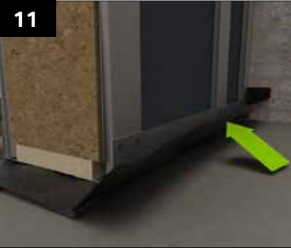
Internally fold up the excess DPC and temporarily fix in place, this can be done with tape or other method.
